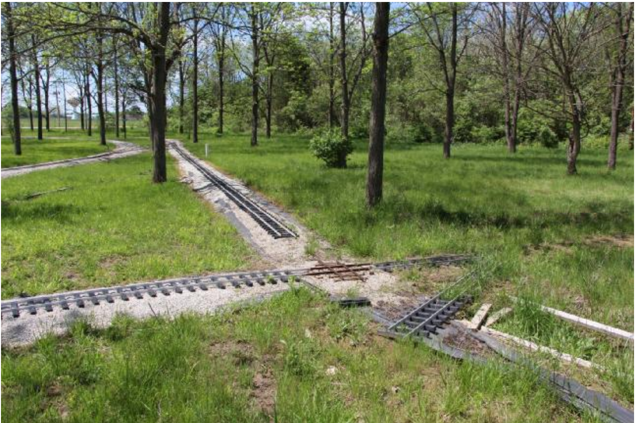
The diamond crossing being installed for Phase 3
